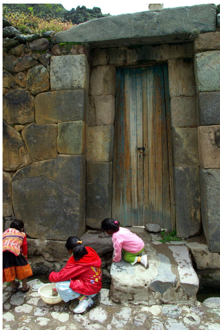
A typical Inca doorway still used in the town. Note the single stone lintel, a sign of importance.
