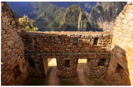
Partially restored Inca building
